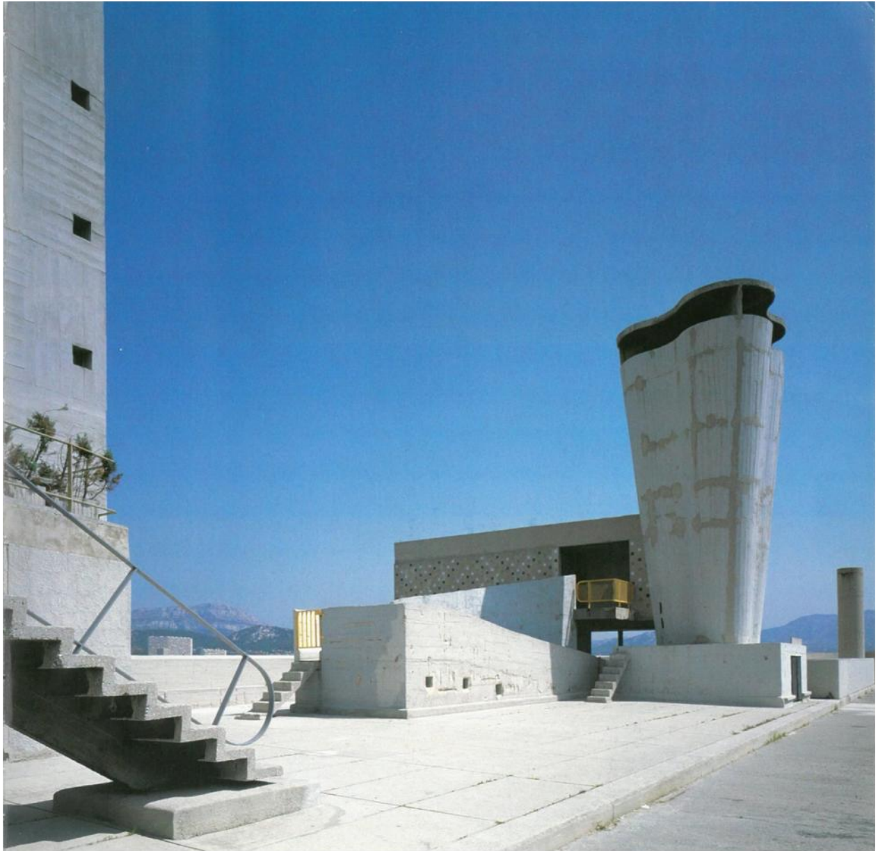
Rooftop and ventilator shaft of the Unité d'Habitation Marseilles. Photo Credit: Peter Cook in Jenkins, David. Unité d'Habitation Marseilles: Le Corbusier (London: Phaidon Press, 1993), 40.
